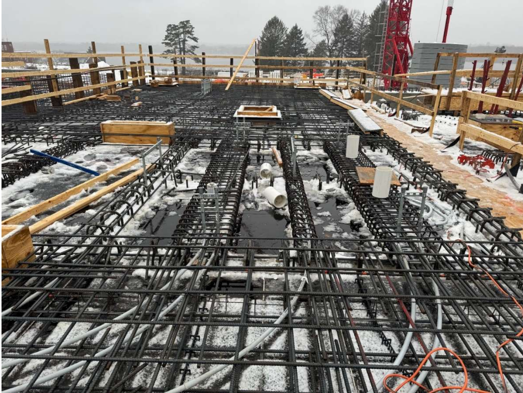
Griffin continued to install in-slab conduits for the rapid mix equipment.
