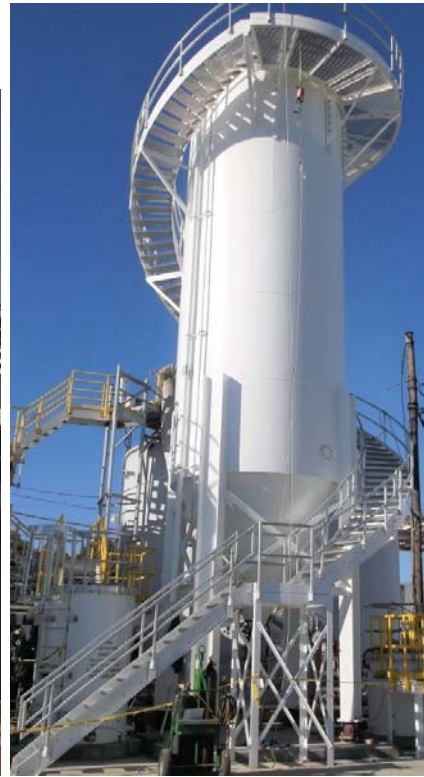
Skirted silo with stairway
