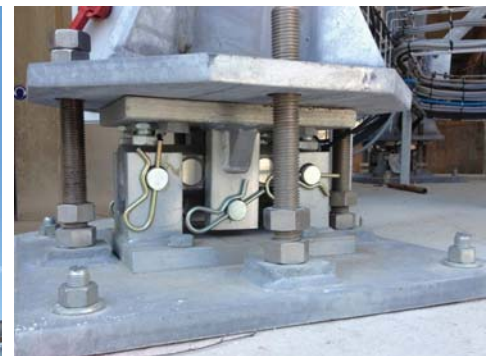
Load cells for skirted silo
