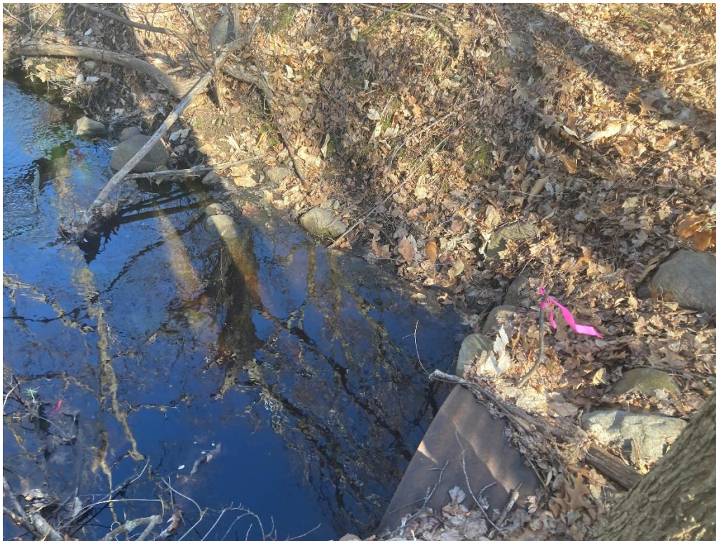
Photo 4: View from above of existing 36-inch corroded culvert and intermittent stream channel.
