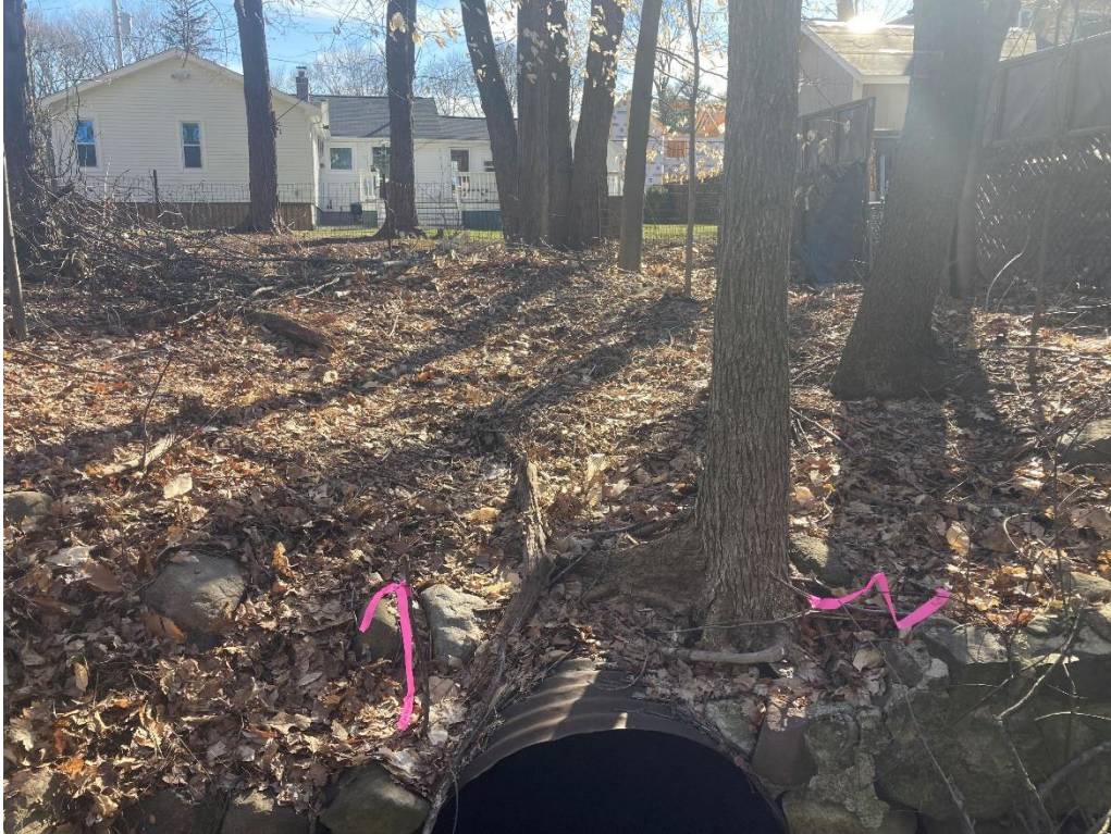
Photo 3: View facing east towards 10 Revere Street, showing the corroded 36-inch culvert.
